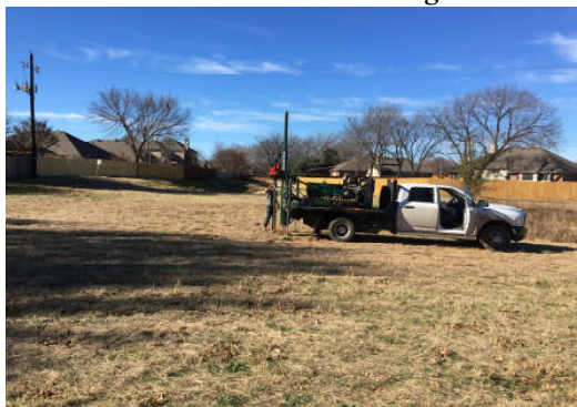
Site Photo 3.1.1 -Looking West
