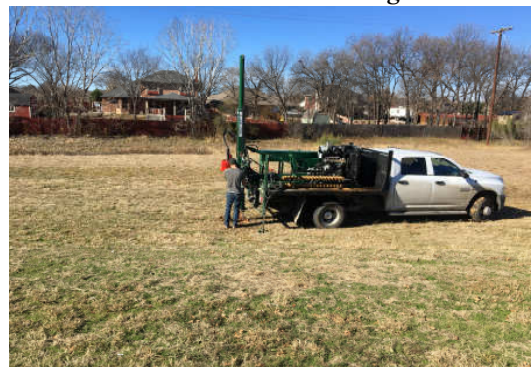
Site Photo 3.1.2 -Looking West
