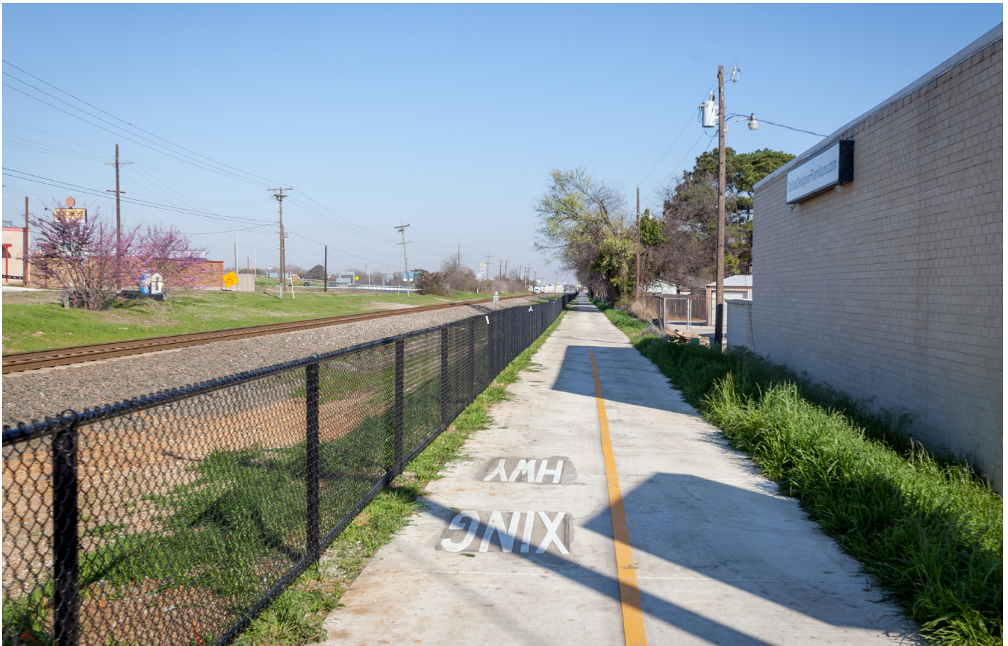
Newly constructed DCTA Rail Trail
