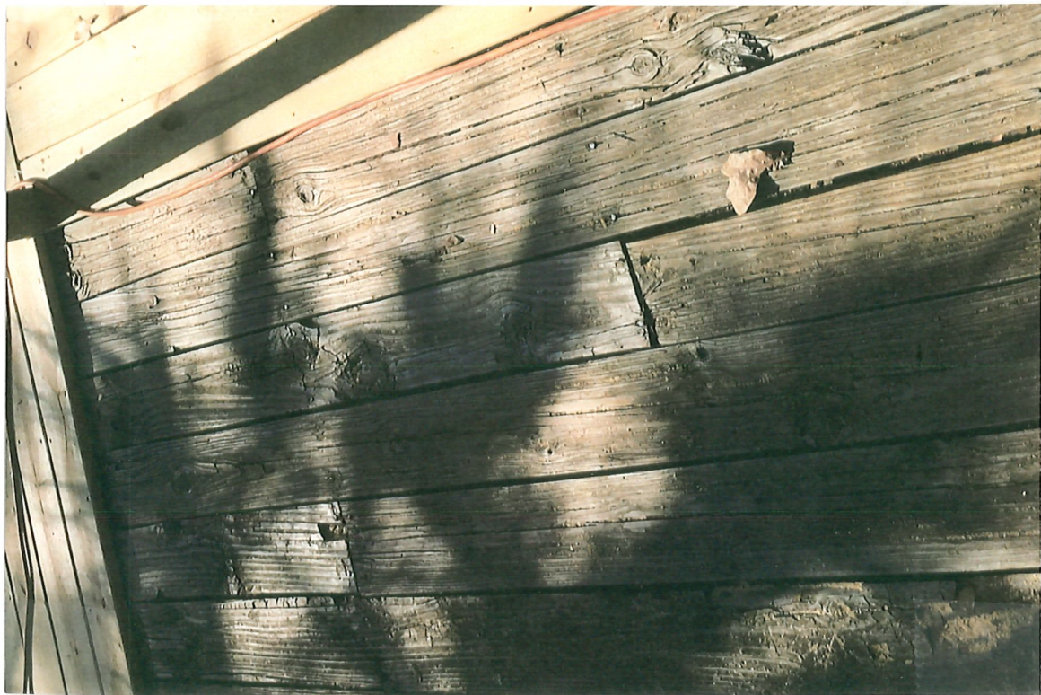
Porch Flooring Boards 2017
