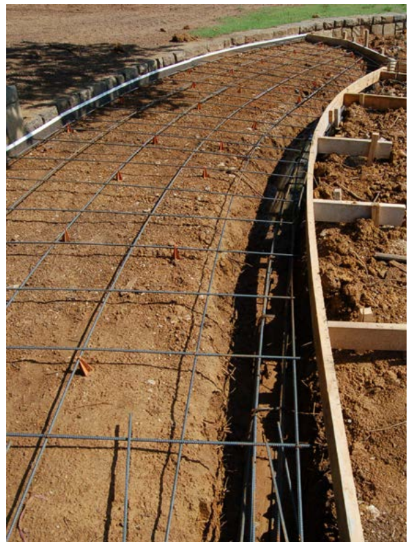
Trail Under Construction
