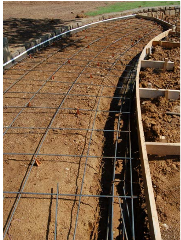
Trail Under Construction
